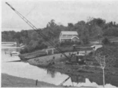
Dredging at Canary-Oriole Bay.
